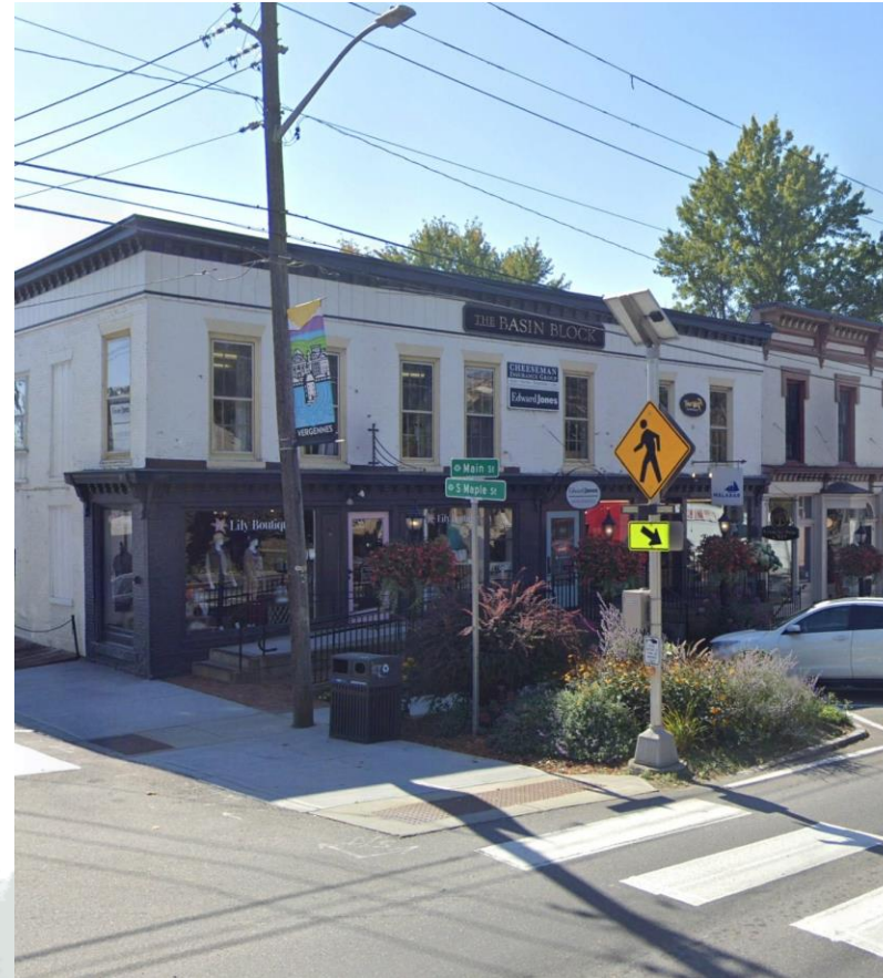
The Basin Block Main Street and Maple Street, Vergennes
