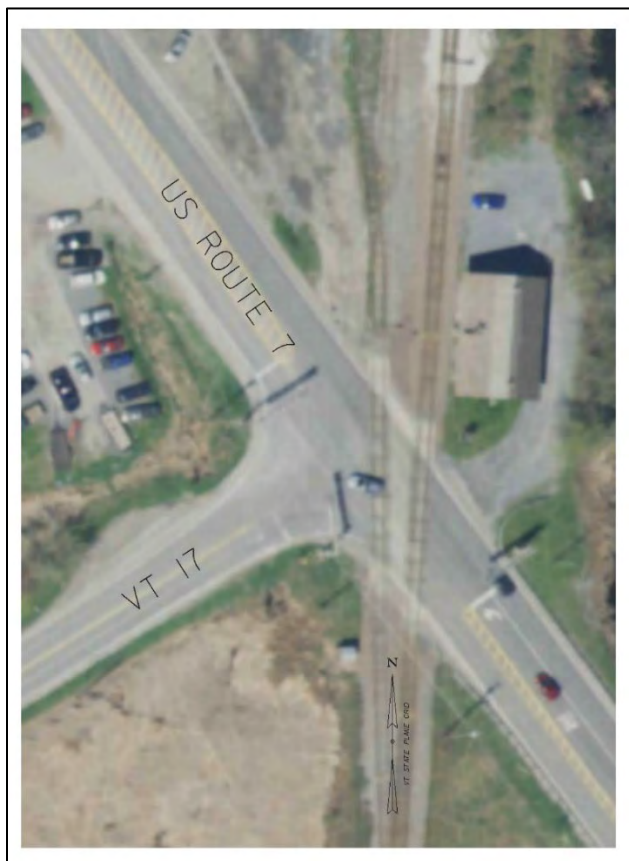
Figure 4-22 VT 17/US 7 Intersection
