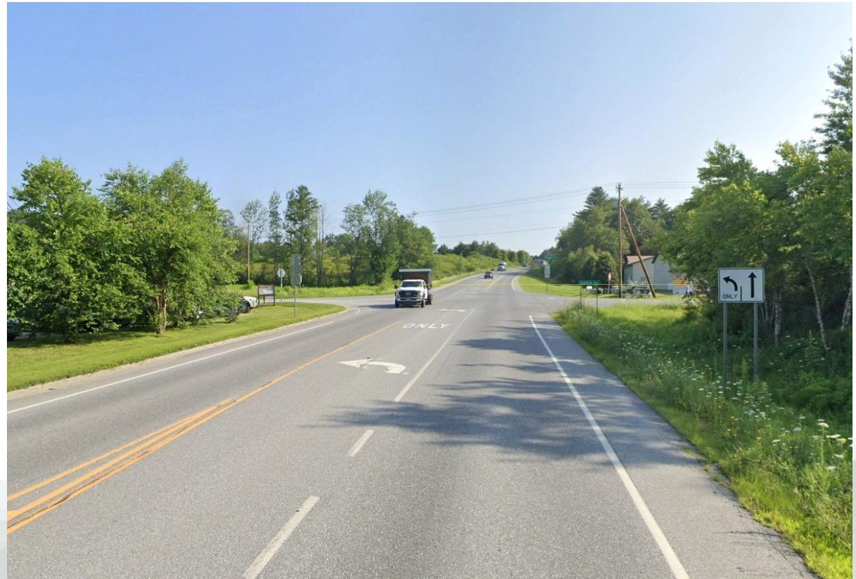
VT 100 intersection with Stafford Avenue (Google Earth)
